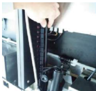
Refit the cover to the conduit
